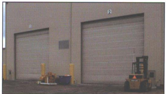
4 - 36' x 34' MEGADOORS are installed at Triton Coal near Wright, Wyoming.
