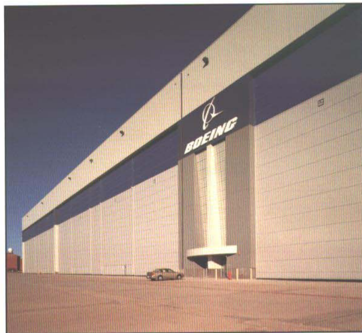
Boeing 747 3-Bay Hangar, Wichita, Kansas; 238' W x 78' H, 258' W x 78' H, 259' W x 78' H., Architect: Gossen, Livingston, Architects, Wichita, Kansas
