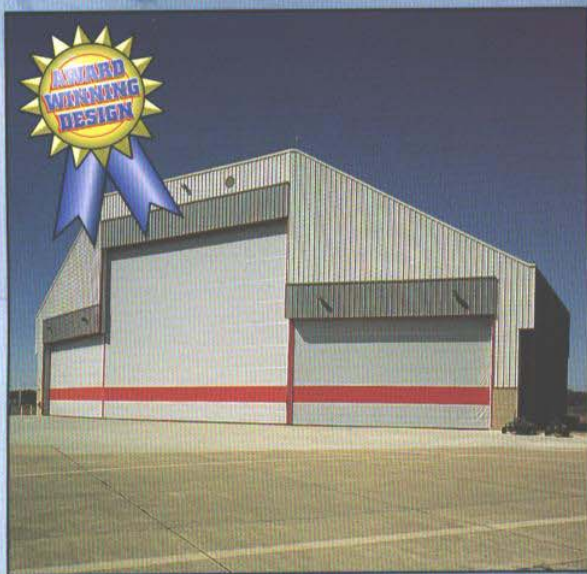
C-141-B/C17-A Fuel System Maintenance/Corrosion Control Hangar for the Tennessee Air National Guard in Memphis, Tennessee. The design by Pickering Firm, Inc., Architects of Memphis was the 1995 Engineering Excellence Grand Award Winner.
