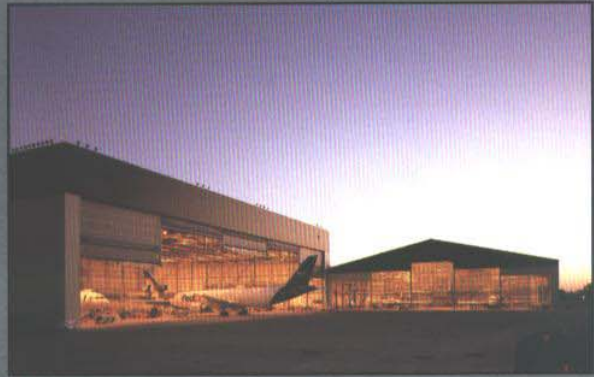
FedEx Heavy Maintenance Facility, Memphis Tennessee Hangar 12 - 384' x 70', Hangar 11 272' x 60'/50'/40' Architect: Frankfurt-Short-Bruza Associates, P.C., Oklahoma City, Oklahoma
