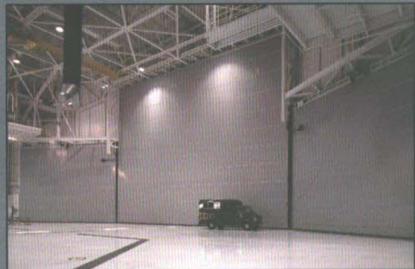
Kansas Air National Guard - B-1 Shaped Hangar Wichita, Kansas, 160' x 27'/46' Doors Architect: McCluggage, Van Sickle & Perry
