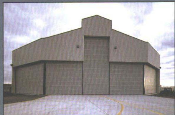
Maine Air National Guard - KC-135 Shaped Hangar Bangor, Maine, 162' x 49'/28'. Architect: Oest Associates, S. Portland, Maine
