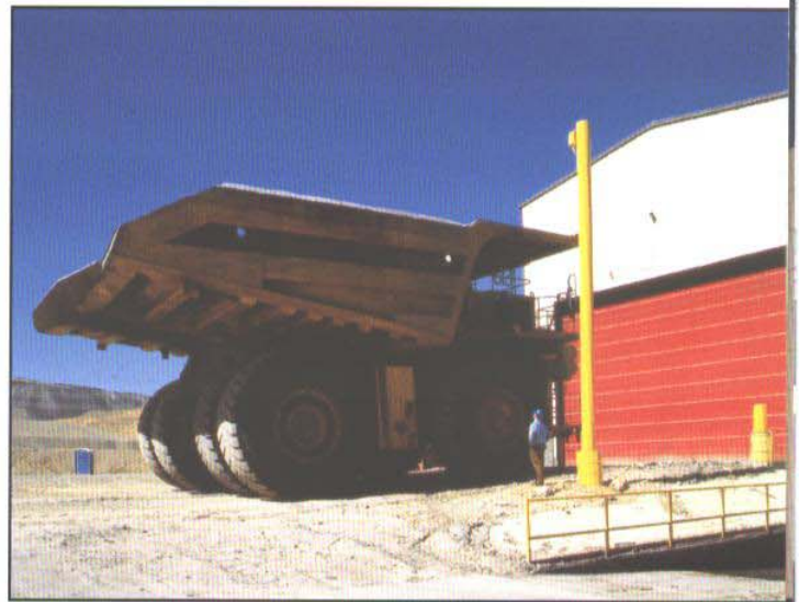
In the dirt and grime of the Barrick Gold Strikes wash bay facility, 2 - 38' x 28' MEGADOORS dependably operate every day.
